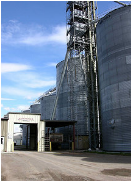
Entrance to the linseed oil facility
