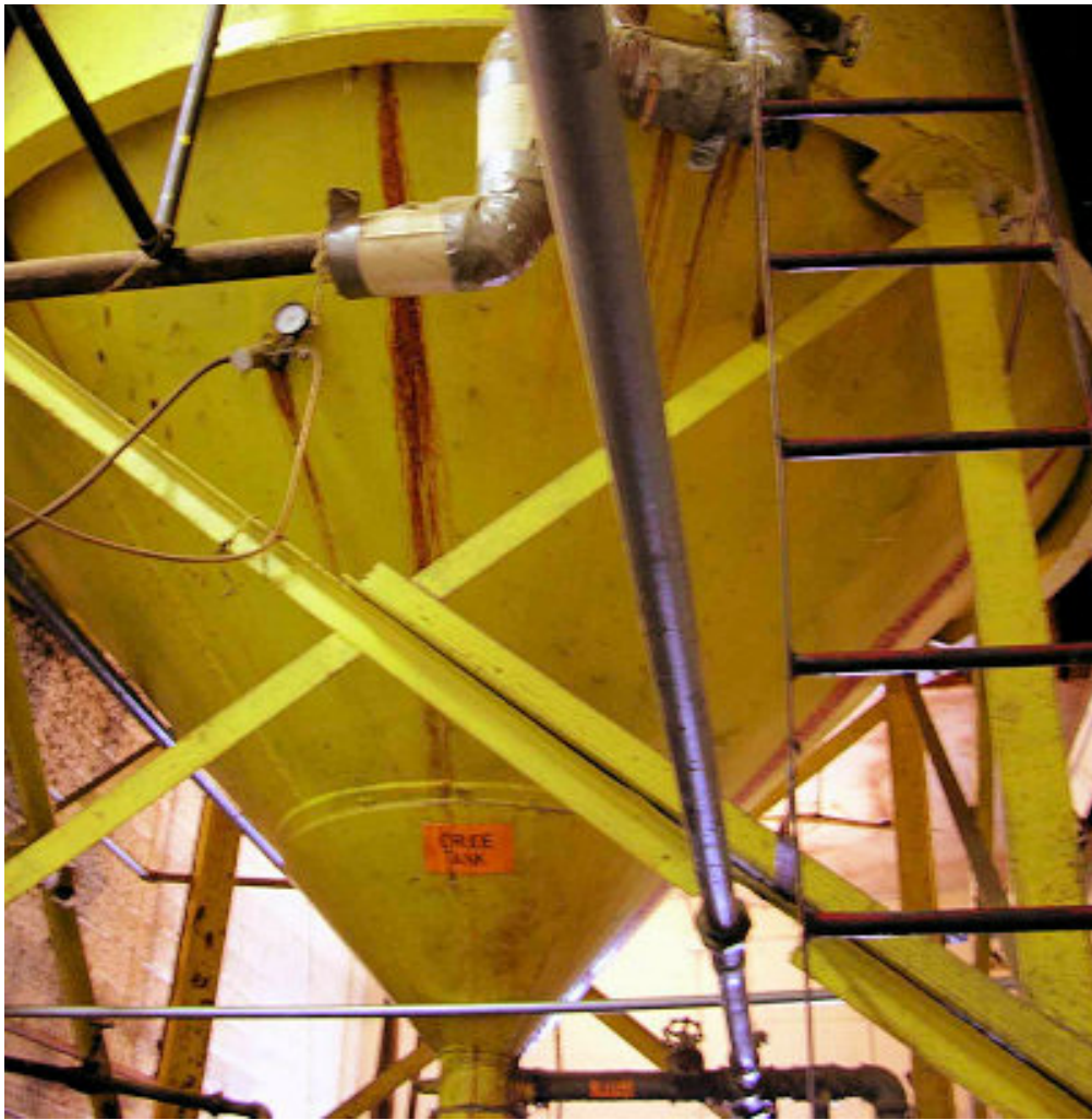
Gravity pulls oil and sediments down through the tank.
